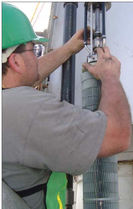
The changeout/installation of SSR catalysts was completed by CPIngredientes plant staff and supervised by Catacel.
