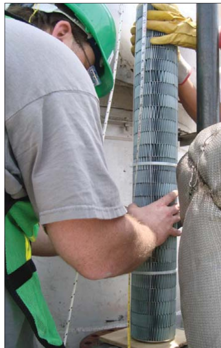
The changeout/installation of SSR catalysts was completed by CPIngredientes plant staff and supervised by Catacel.
